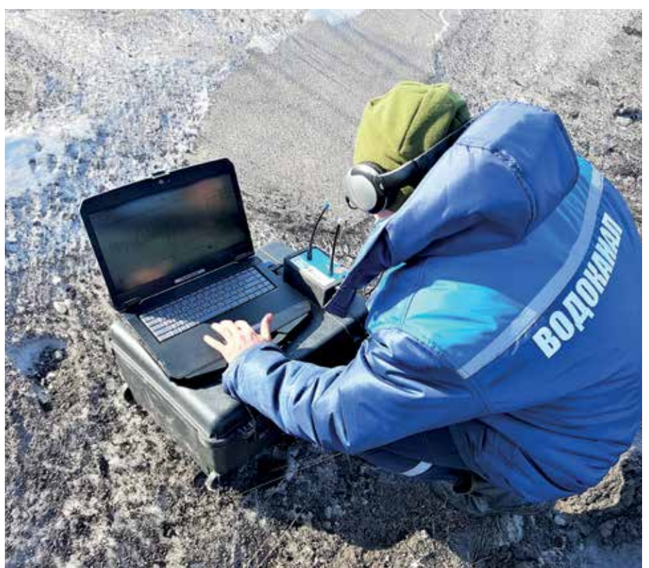
Listening for leaks
